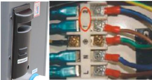
**Water pump wiring**
